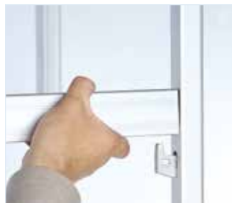
schuif de dwarsverbinders over de inhaakdragers
